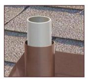
Vent pipe must extend 2" to 5" above base sleeve to allow for roof expansion and contraction. Cut off excess pipe above 5".
