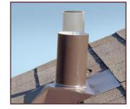
Place new vent pipe flange next to vent pipe and visually check pitch alignment.
