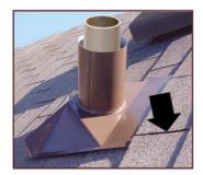
Upper flat section of flange must be completely covered. If necessary, rotate under two rows of shingles and trim shingles to fit.
