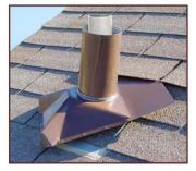
Place the vent flange over the vent pipe and rotate into position under one or more rows of shingles.
