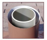
Visually check the base sleeve centered around the vent pipe for equal air circulation
