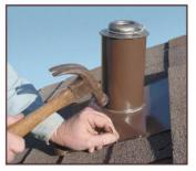
Use embossed guides around perimeter of the base flashing to securely nail the base to the roof.
