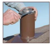
Slide the top sleeve over the base cylinder until the lead seal fits tightly on the vent pipe.
